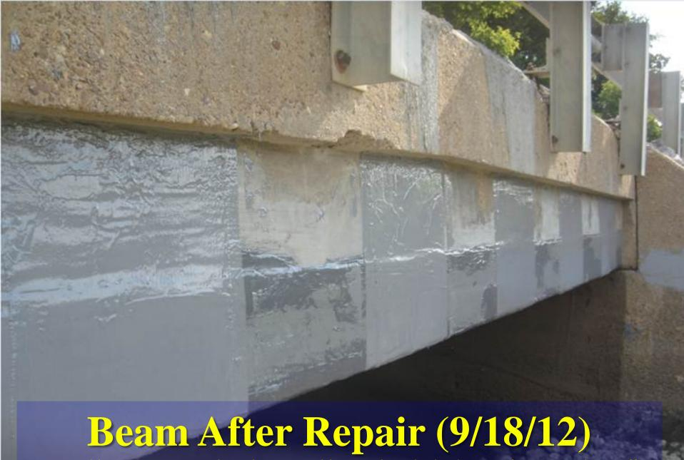
(Repaired beam is stronger than the original beam when the bridge was first opened to traffic)
